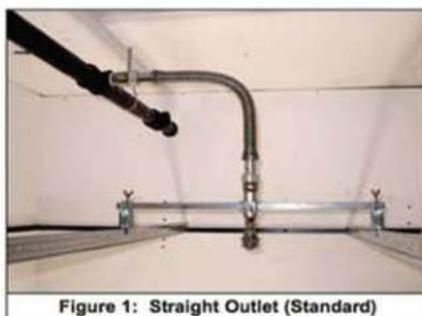
Figure 1: Straight Outlet (Standard)
