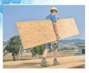
OSB stands for "Oriented Strand Board" and is a wood-based product made from thin veneer strands that are bonded together with a synthetic resin. This OSB consists of three cross-oriented layers with the surface of the board formed from strands oriented along the length of the board and the core strands arranged in cross orientation. This crosswise orientation of the individual layers achieves a high level of dimensional stability and an excellent mechanical performance.
