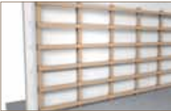
horizontal support battening = installation CP vertical
